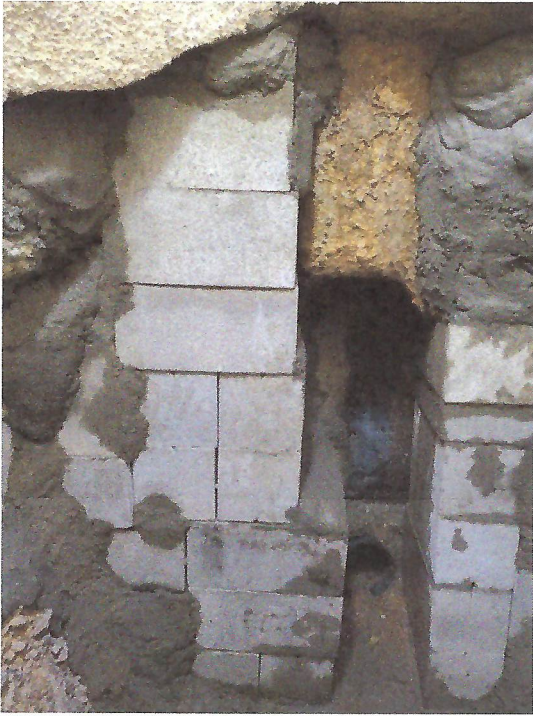
Manhole #2: Rebuilt Back Wall with Concrete Blocks to Fill in Voids and Restore Structural Integrity
