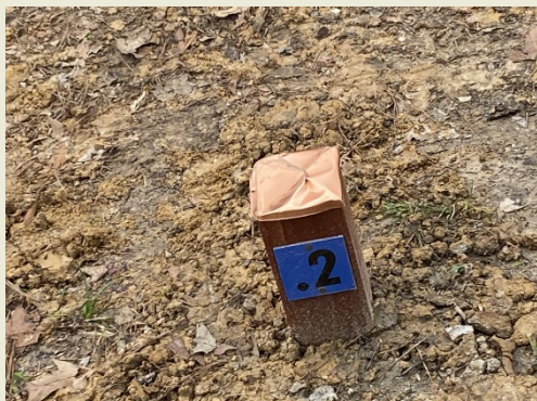
All 20 newly installed mile markers have been damaged.
